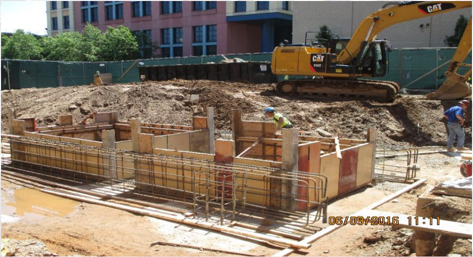
Footing for New Staircase
