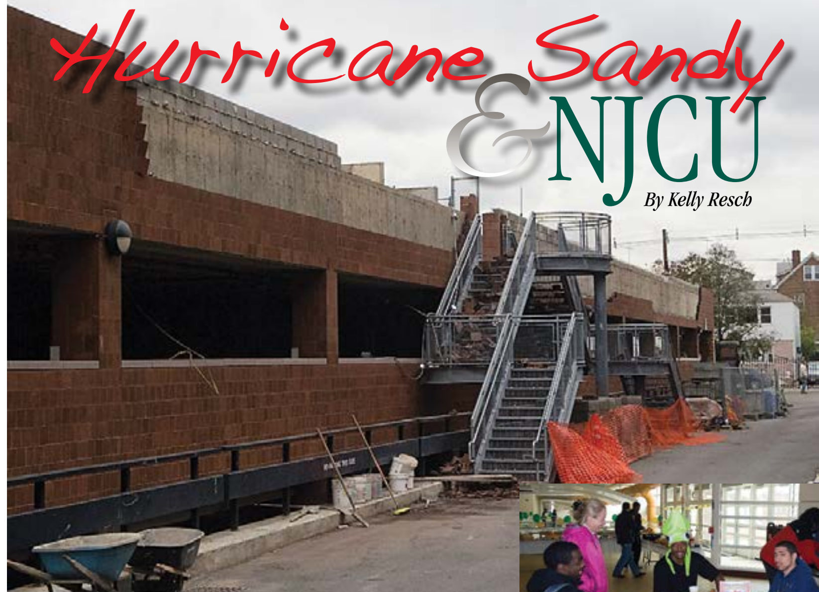
Winds from Hurricane Sandy ripped brick facing from the outer wall of the Michael B. Gilligan Student Union.
