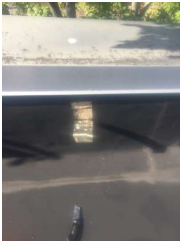
Parapet wall flashing
